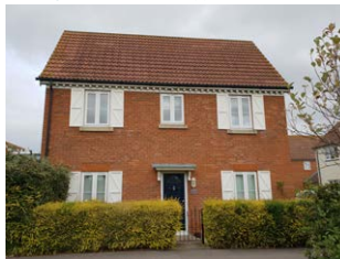
Existing detached house opposite
